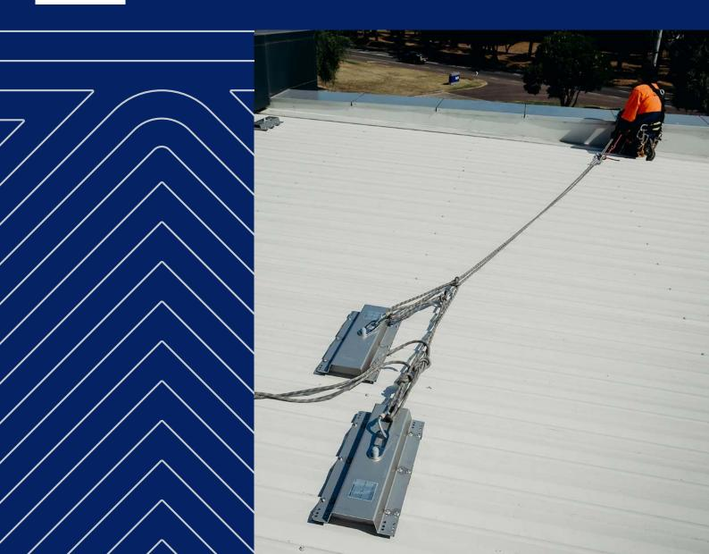
The Kattsafe top mount rope access anchor is designed for fast installation and ultimate strength, for abseil workers.
