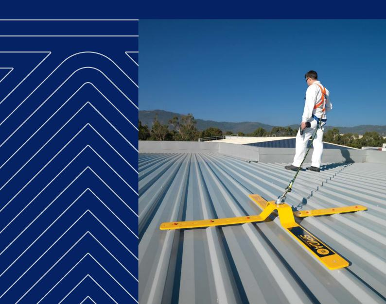
Temporary anchor for an easy and cost-effective fall arrest solution for maintenance workers regularly accessing unprotected roofs.
