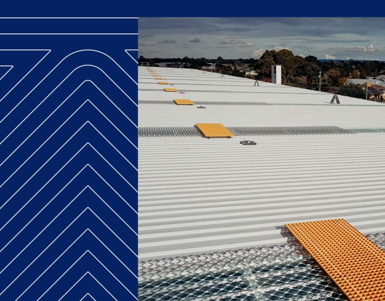
Kattsafe's skylight protectors are lightweight, high strength aluminium protection to cover skylights for personell safety on the roof.
